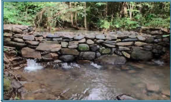
Loose boulder check dams and Gabion Check dam
