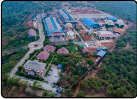
Integrated Solid Waste Management Facility at Saligao
