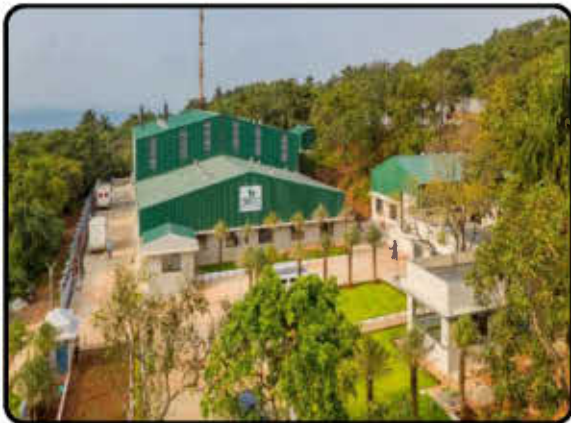
Common Biomedical Waste Treatment Facility at Kundaim
