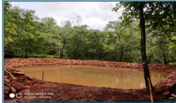
Water Retaining Sunken Pond
