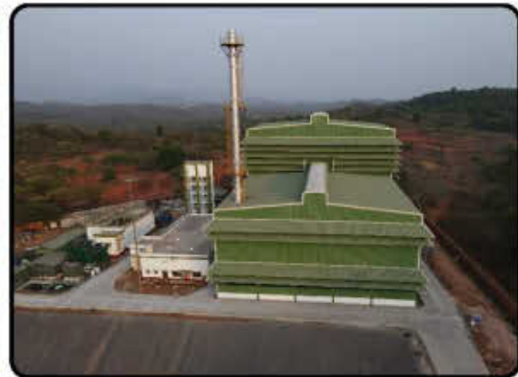
Common Hazardous Waste Treatment, Storage and Disposal Facility at Pissurle
