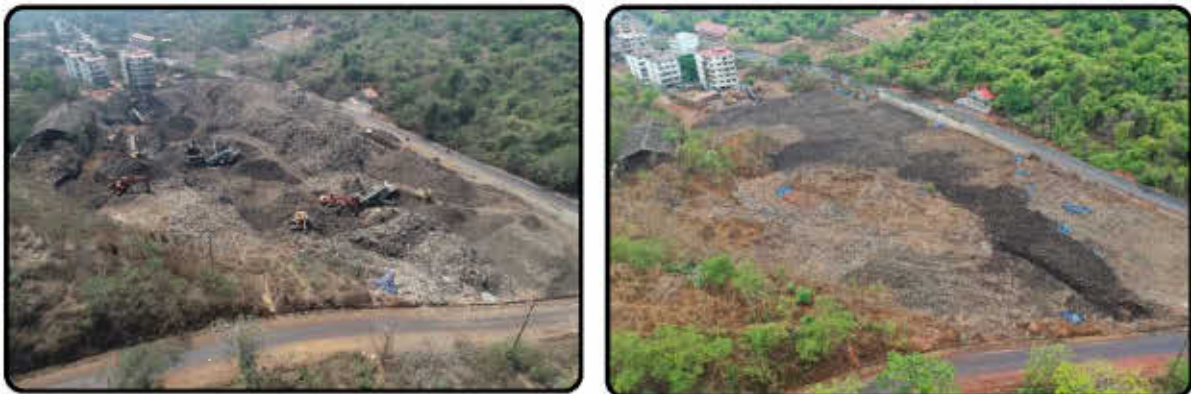
Remediation of legacy dumpsites Before After
