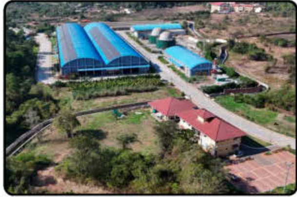
Integrated Solid Waste Management Facility at Cacora
