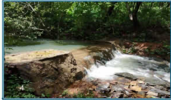
Cement mortar check dams
